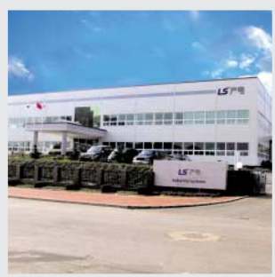
Dalian Plant (China)
