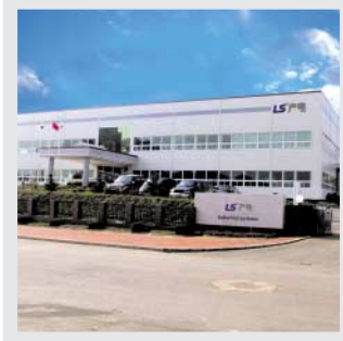
Dalian Plant (China)
